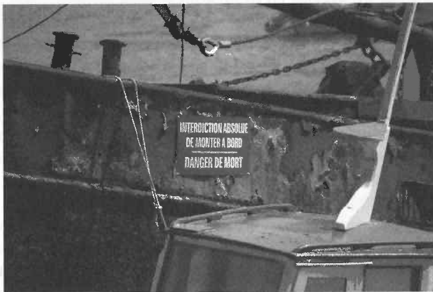
18.5 A warning of the safety hazard caused by a derelict steel ship (photograph by Ken Wittamore).
