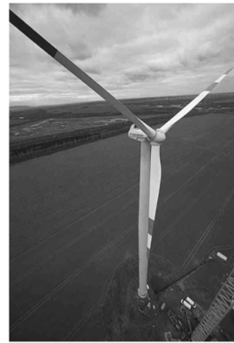
Fig. 8 The 40 m radius AL40 carbon–wood epoxy wind turbine blade
